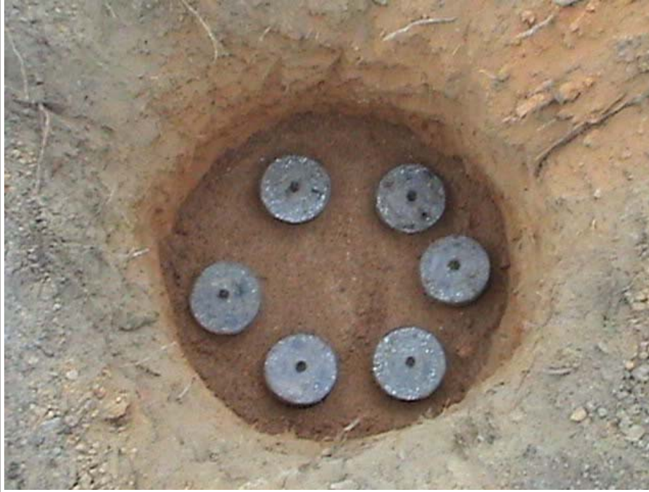
Hole dug, next template placed over quartz points to centre Tb;s
